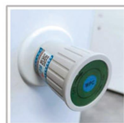
Water Supply Flow Control Valve
